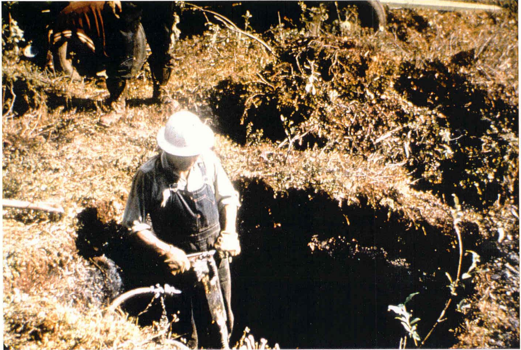
Hank Johnson, digging in permafrost Inuvik, <1960.
