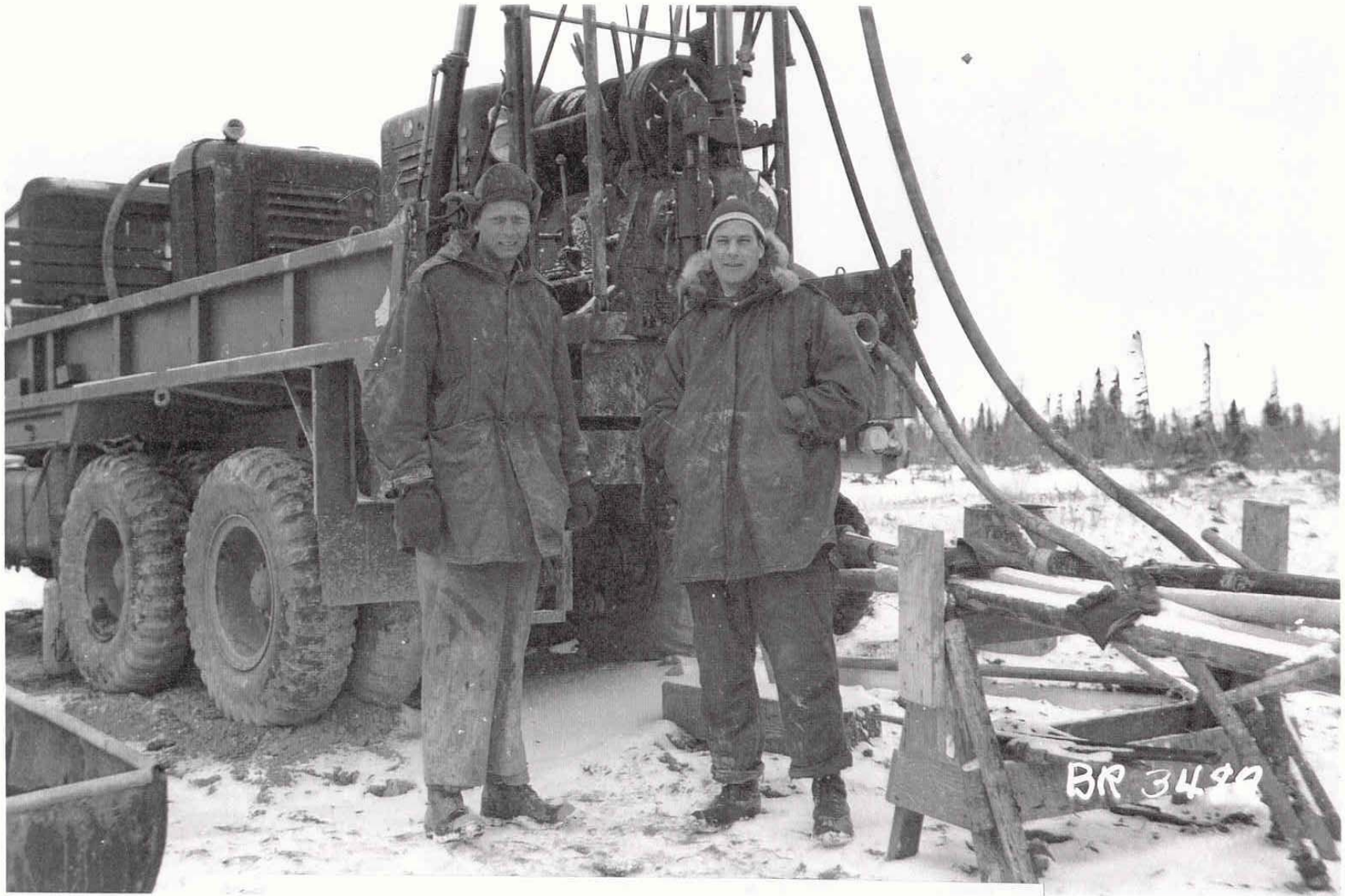
Hank Johnston with Bob Lang, SIPRE, conducting drilling tests in frozen ground.
