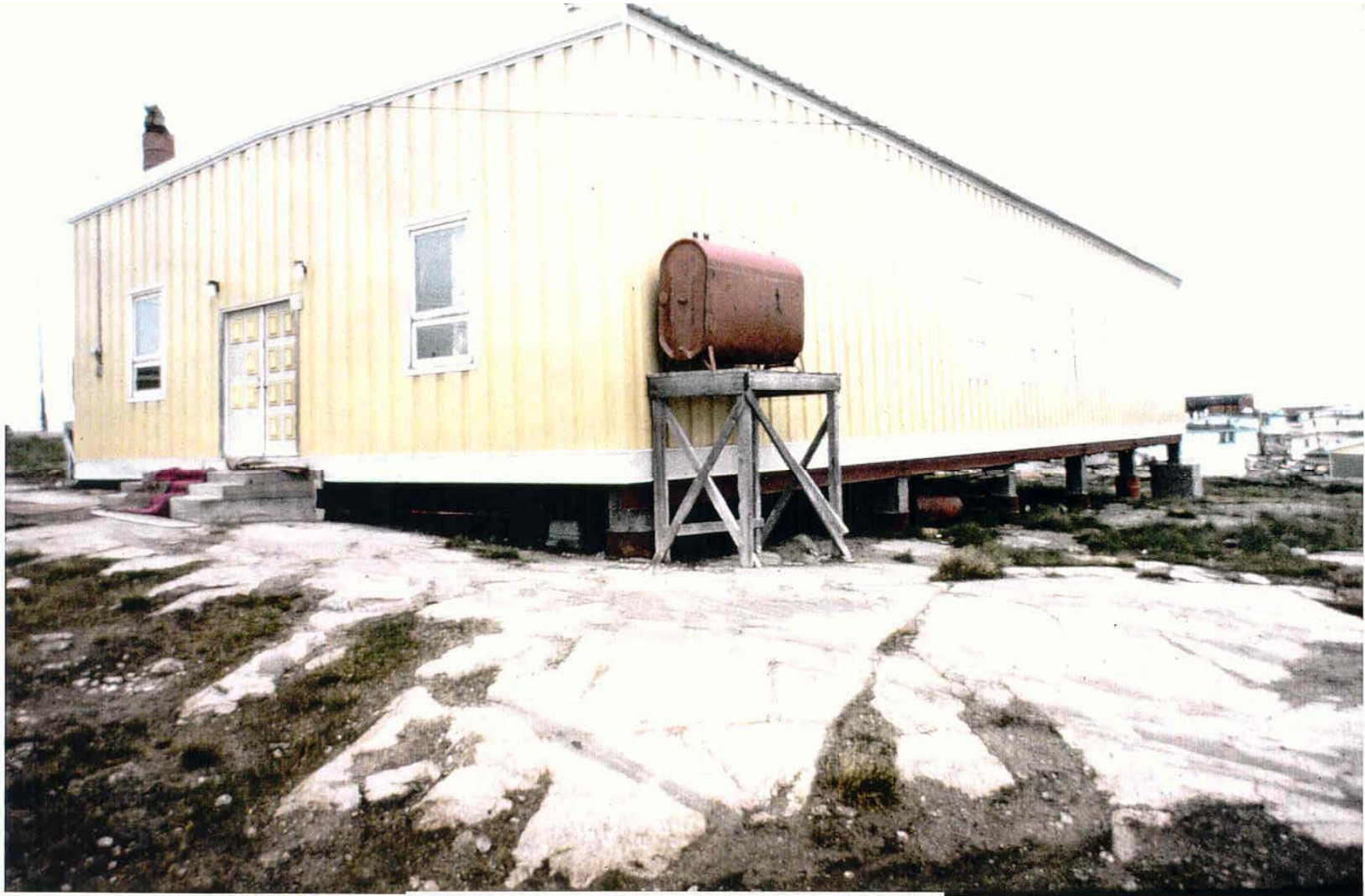
Iqaluit, NWT. "Permafrost Foundations"
