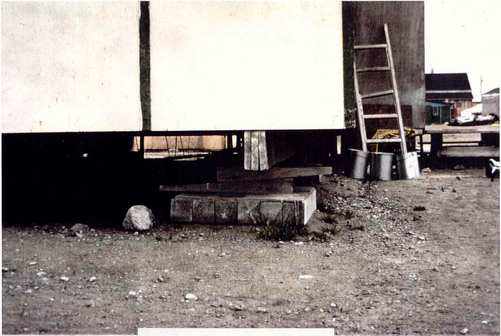
Iqaluit, NWT. "Permafrost Foundations"
