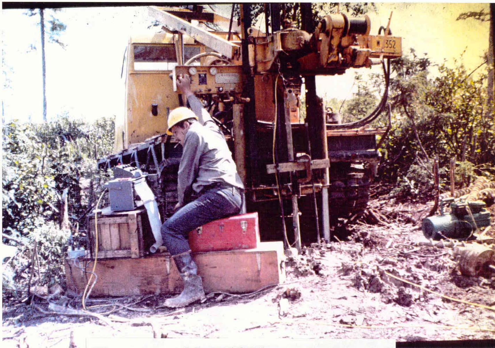
Thompson, Man. 1975. CPT in permafrost. (Ladanyi, Arteau, Paquin)
