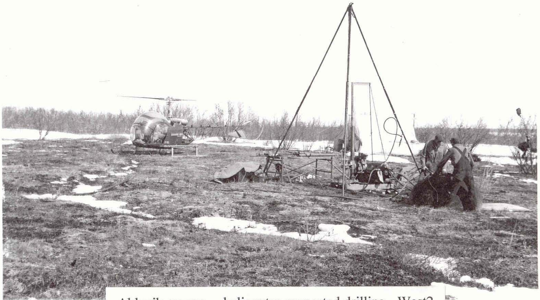
Aklavik survey - helicopter supported drilling - West2 site (Hank Johnston)
