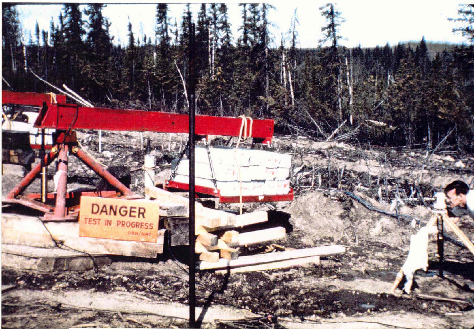
Thompson, Man. 1971. Anchor Tests in permafrost (Hank Johnston & Co.)
