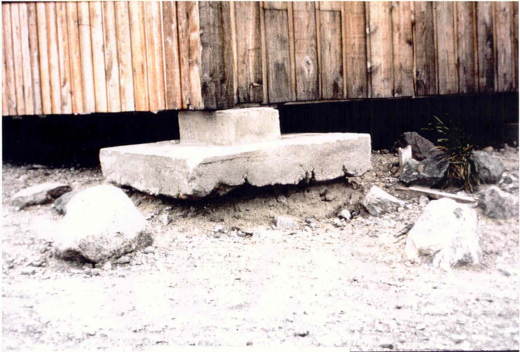
Iqaluit, NWT. "Permafrost Foundations"
