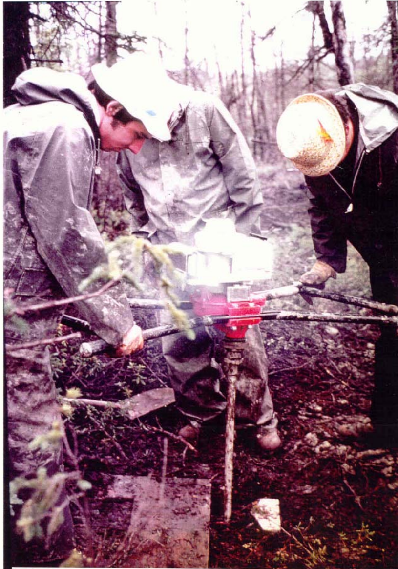
Thompson, Man. 1975. CPT in permafrost. (Ladanyi, Arteau, Paquin)
